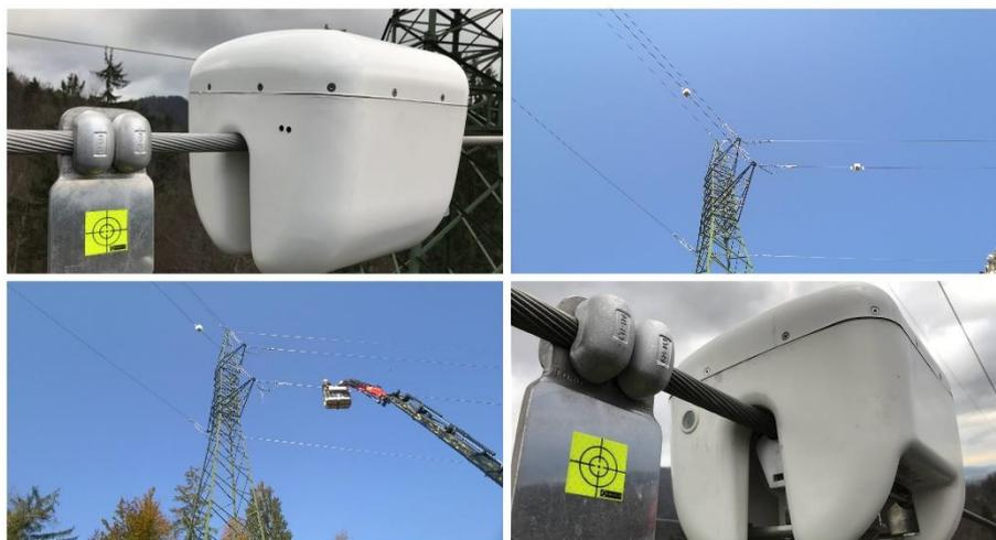
*Figure 1 – ELJ experts are installing OTLM devices on Kleče – Logatec line*
